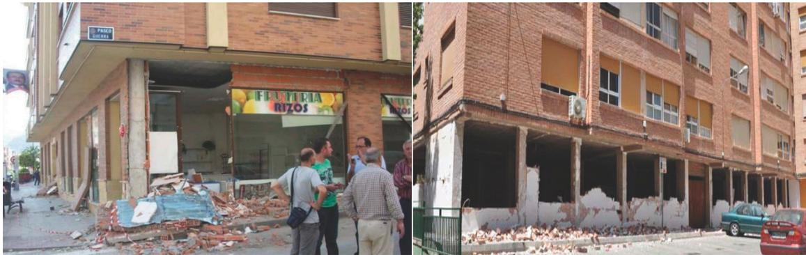
Figure 3. Examples of the soft story phenomena that occurred in Lorca in 2011 after the quake.
