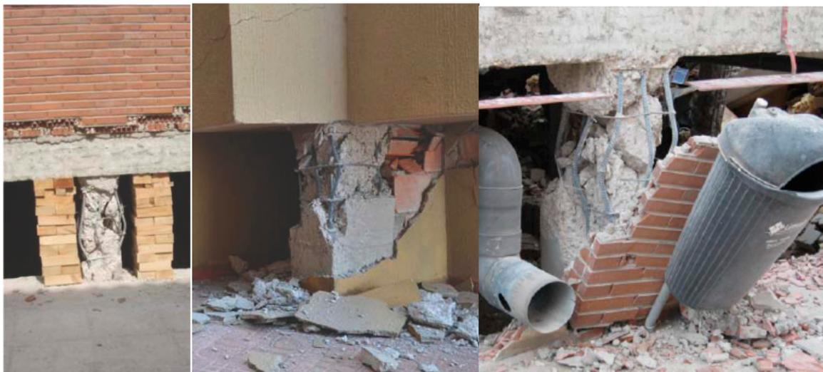
Figure 4. Effect of short columns in different buildings of the city of Lorca after the quake.
