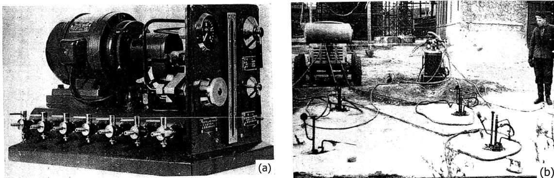
**Figure 2.** Photos of the ground heating equipment and application proposed by Litvinov [22]. (a) The equipment for mixing fossil fuel and air; (b) a photo of the construction the soil heating method.
