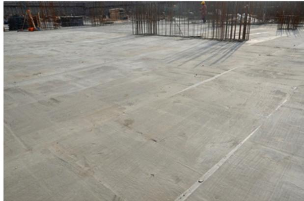
Figure 16. Crack-free surface of the mass concrete foundation slab.
