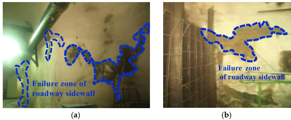
**Figure 2.** Failure zone of the sidewall: (a) Middle-upper part of roadway sidewall; (b) Middle-lower part of roadway sidewall.
