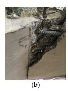
**Figure 10.** Damage to bridge deck slabs at various locations. (a) Damage on the slab side. (b) Damage at variable section locations.
