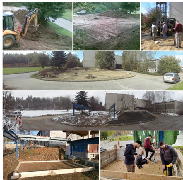
Figure 2. Construction of the Scientific Research Workplace of the Faculty of Civil Engineering at the University of Žilina and measurements of the quality of the clay subgrade.
