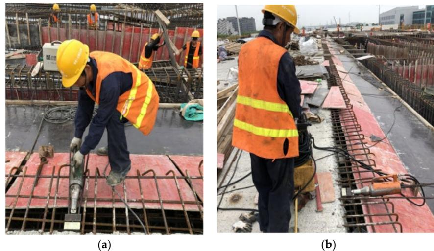
**Figure 13.** Application at construction site: (a) jack installation, and (b) tensioning operation.
