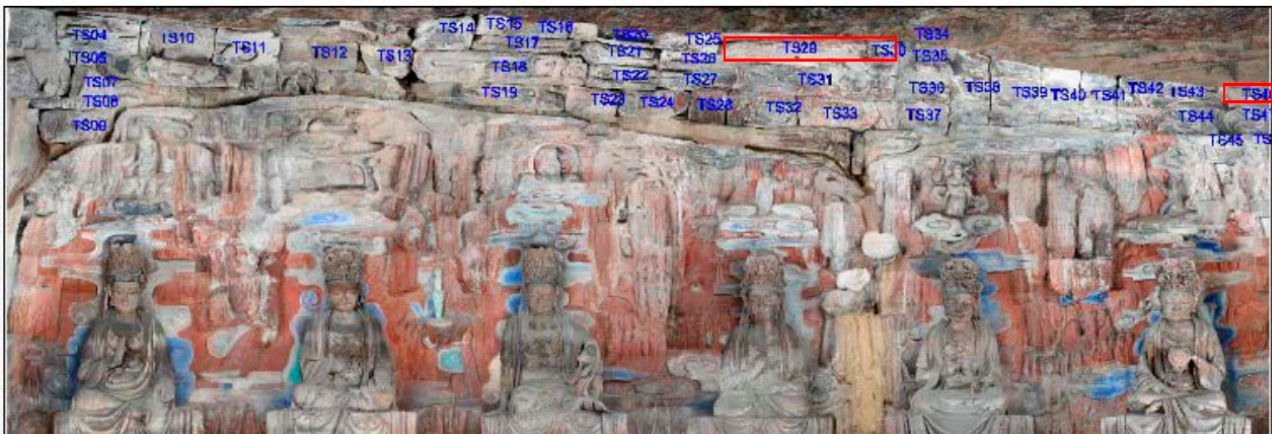
Figure 15. Characteristic points of broken slates and destabilization warning points.
