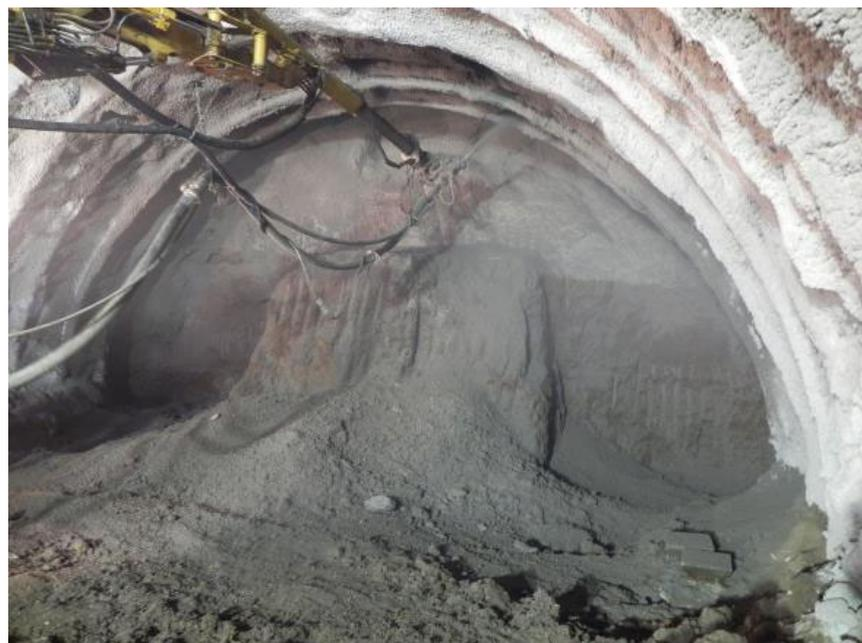
**Figure 39.** Stabilization of the excavation face south portal.
