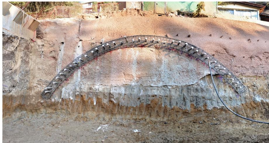
**Figure 4.** Micropiles umbrella with reinforced steel structure in the south portal of the tunnel.
