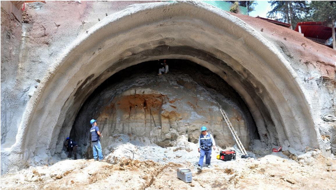
**Figure 27.** Detail of the excavation of the left tube of the South Portal, where there was the least coverage (8 m).
