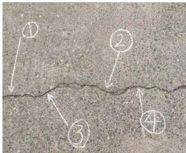
Figure 14. The measured selected position (①, ②, ③, and ④ represent the locations of four crack measurements).
