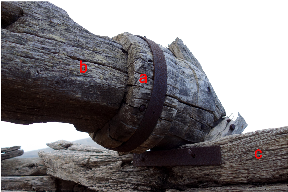
Figure 9. “Violas” (a), found at the windshaft (b), and antixono (c).
