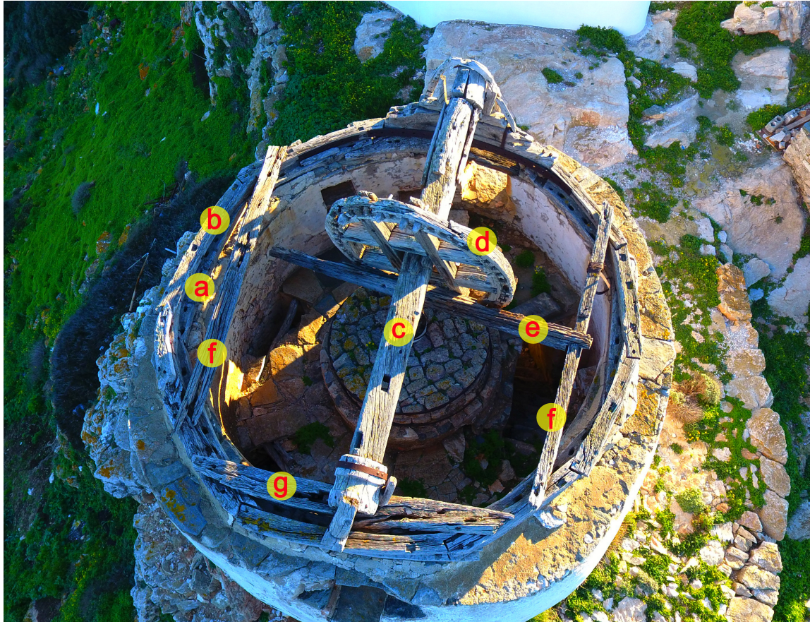
Figure 1. Main wooden parts of the windmill mechanism (a. “katoplakes”, b. “panarika”, c. windshaft, d. wheel, e. “zigos”, f. “bratsolia”, g. “antixono”).
