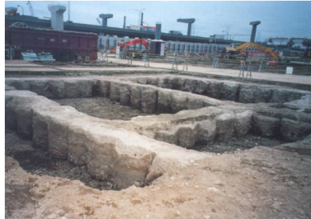
Figure 9. Grid-type DM-improved ground.
