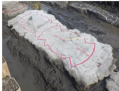
Figure 10. Rectangular-shaped stabilized soil column constructed via jet grouting method (courtesy of the Chemical Grouting Co., Ltd.).
