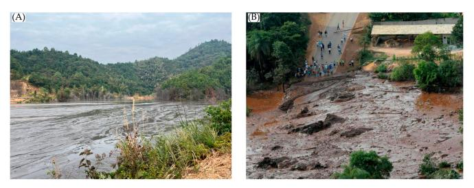
Figure 6. (A) Tailing Pond; (B) Brazilian iron ore tailings dam break accident in 2019.
