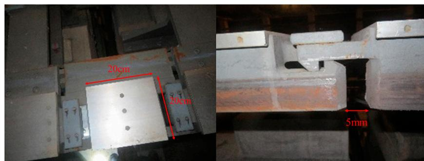
**Figure 7.** Rail expansion joint photos.
