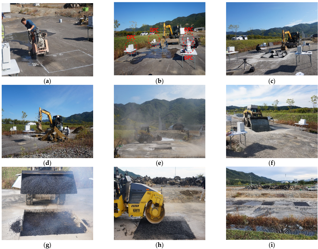
Figure 3. First field test. (a) Cutting, (b) breaking, (c) removal, (d) excavation, (e) site sweeping, (f) restoration, (g) asphalt laying, (h) compaction, and (i) completed asphalt pavement (Sections 4–6).
