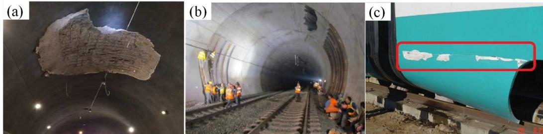
**Figure 1.** Impact on driving safety of spalling blocks comprising a tunnel lining. (a) Flaky block; (b) blocky block; (c) The falling block collided with the train.
