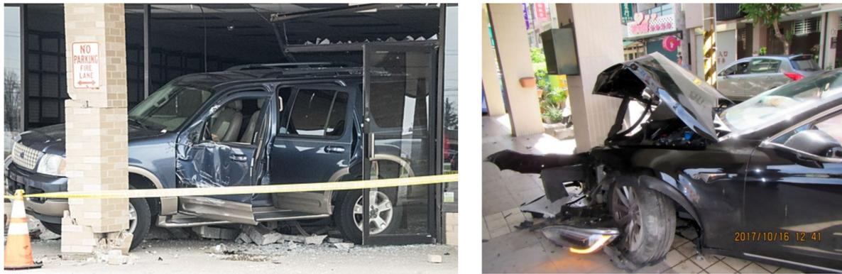
**Figure 1.** Cars crashed into RC columns on the ground floor [7].
