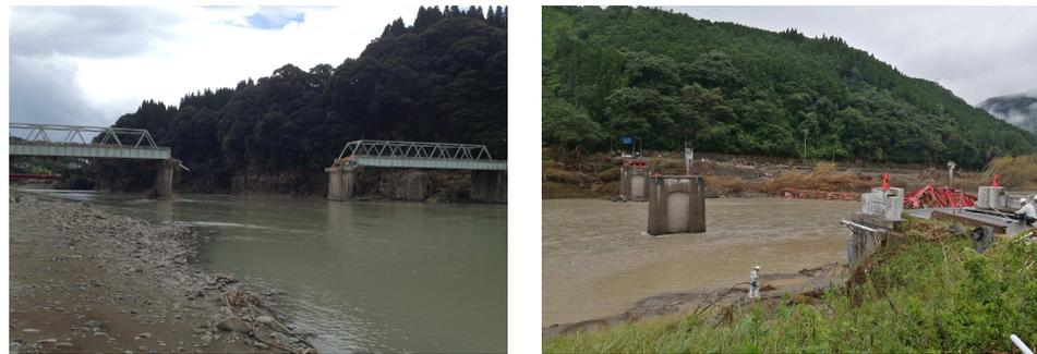
**Figure 1.** Collapsed bridges due to flooding in Kumamoto, Japan (July 2020).
