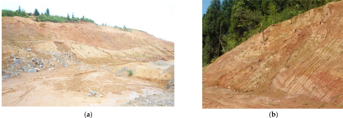
Figure 2. View of the high liquid limited slope: (a) slope panorama, (b) landslide part.
