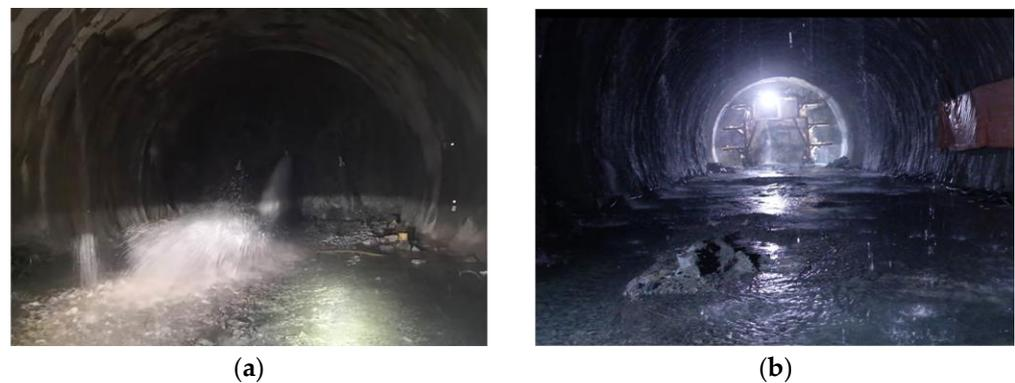
**Figure 3.** Water gushing at the tunnel face. (a) Tunnel face; (b) the vicinity of tunnel face.
