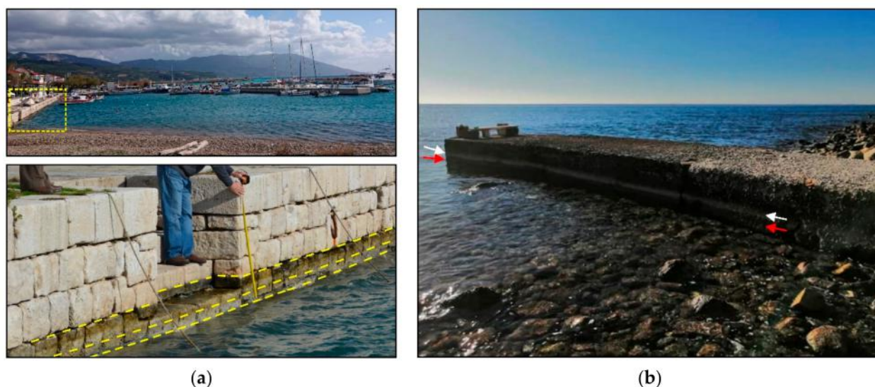
Figure 11. (a) The marina of Marathokampos, which was uplifted not only by the mainshock on 30 October 2020, but also by an aftershock on January 20, 2021. (b) The uplift from the mainshock and the aftershock was also imprinted on a small jetty of the Campos village, located west of Marathokampos village. The white arrow points to the uplift induced by the mainshock and the red ones to the uplift by the aftershock.
