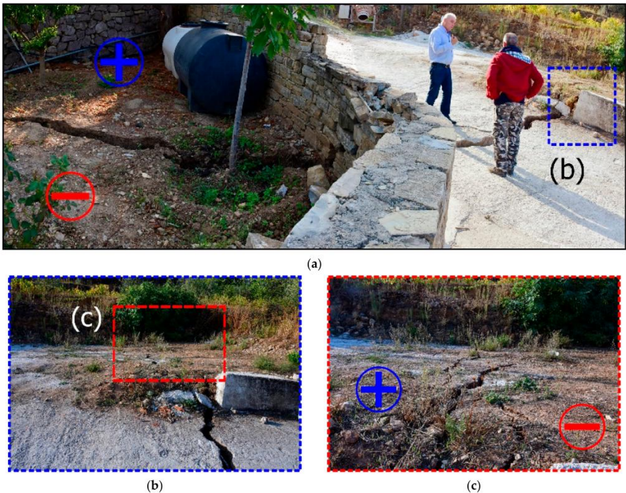
Figure 16. Coseismic surface ruptures in the area between the Vrysses village in the west and the Kontakaeika village in the east. They were continuous affecting a perimeter wall, a concrete road (a) and its adjacent slope (b,c). The red symbol (−) corresponds to the subsided block, while the green symbol (+) corresponds to the uplifted block.
