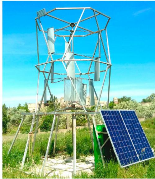
**Figure 11.** Combined wind-solar power plant with a three-section Darier rotor and two photoelectric modules (Sevastopol, SRC «Horizont»).
