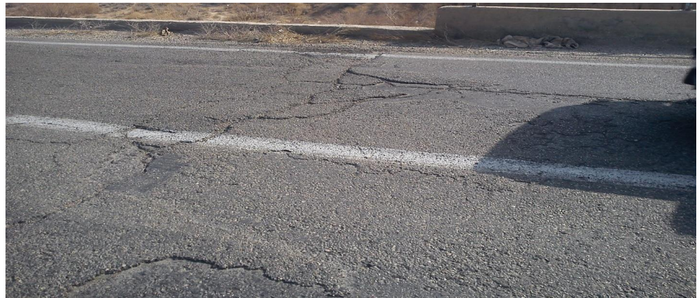
Figure 19. Condition of pavement distresses in bridge NO. 4.
