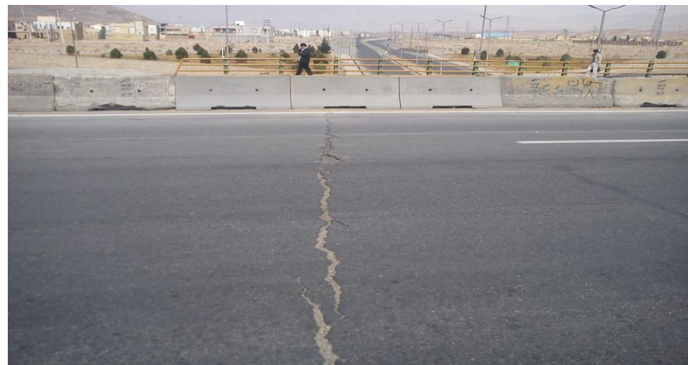
Figure 8. The pavement condition in the bridge No. 1.
