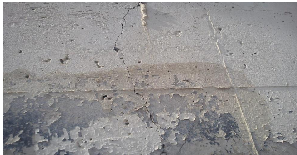
Figure 7. An example of minor cracking in the wall of the bridge No. 1.
