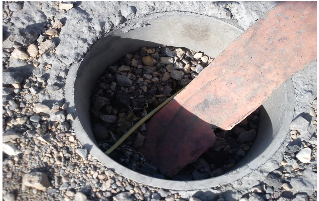
Figure 11. An example of block in the facilities of drainage system (bridge No. 2).
