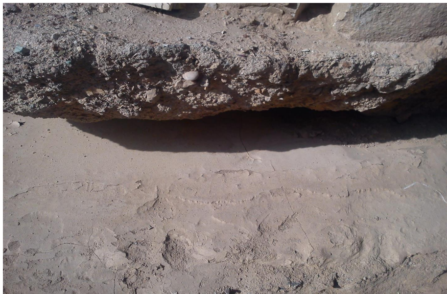
Figure 22. Bridge scour in bridge No. 5.
