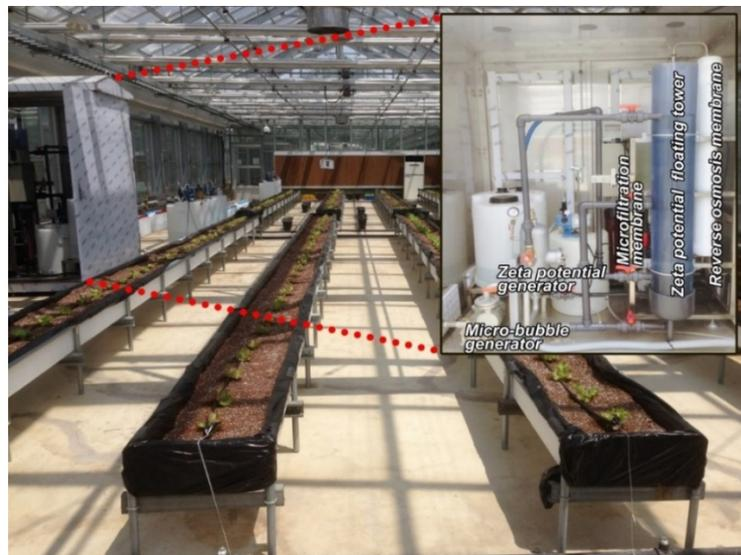
**Figure 1.** Small-scale brackish water desalination (BWD) system installed in the experimental site and experimental plots planted with lettuce.
