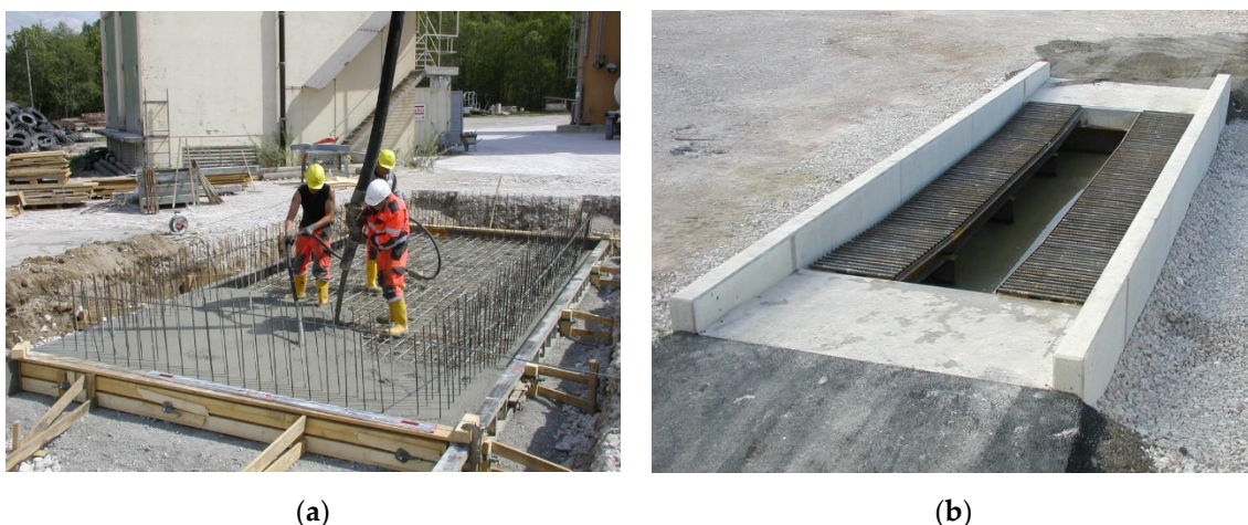
Figure 11. Test track construction using (1) CEM V/A (S-V) 32.5 R using a cement content of 400 kg/m 3 and a water-binder ratio of 0.45 during (a) concreting work and (b) after finishing the construction.
