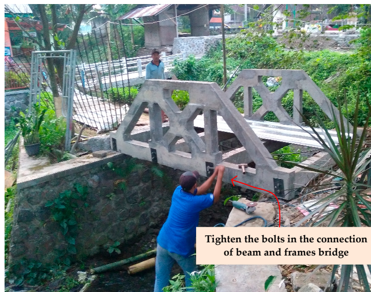
(c) Precast bridge frames
