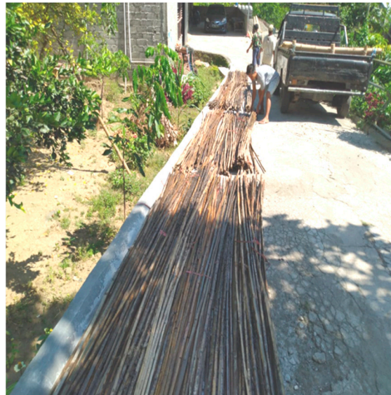
Figure 4. Drying bamboo in free air.
