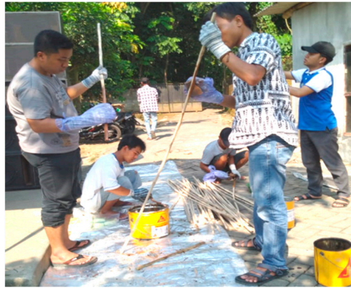
Figure 6. Give a waterproof coating.
