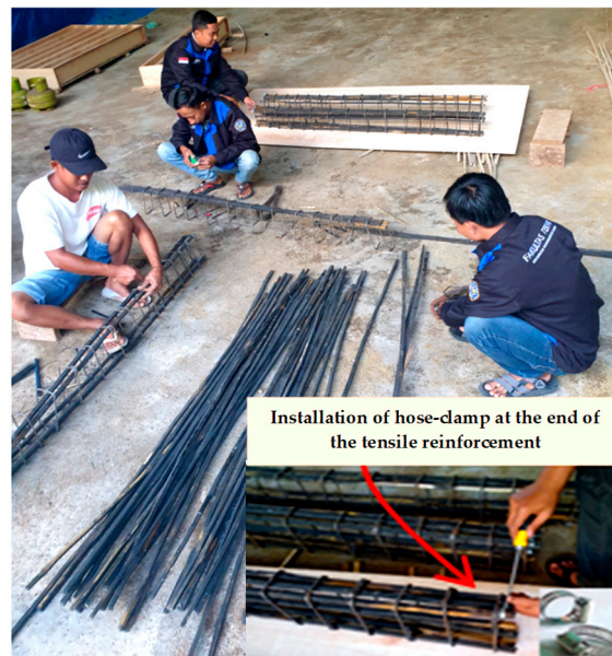
Figure 8. Stringing the bamboo reinforcement.
