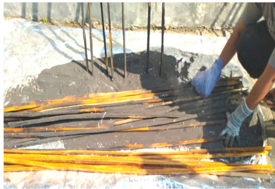
Figure 7. Sand sprinkling on bamboo reinforcement.
