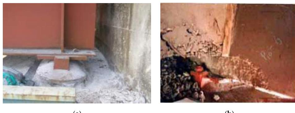
**Figure 6.** Damage of line bearings: (a) the line bearing type for replacement [5]; (b) the corroded top plate of the line bearing [4].
