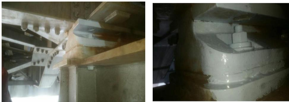
Figure 5. Installation status of the Yeongjong Grand Bridge line bearings.
