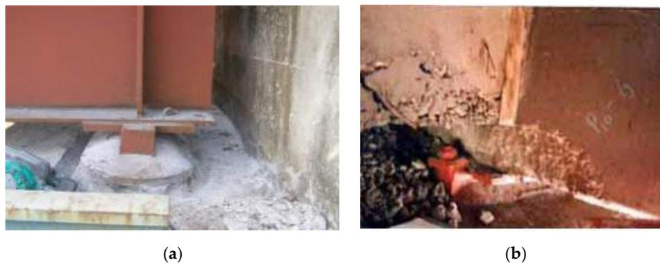
Figure 6. Damage of line bearings: (a) the line bearing type for replacement [5]; (b) the corroded top plate of the line bearing [4].
