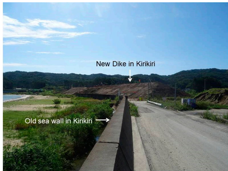
Figure 8. The new dyke in Kirikiri was rebuilt to a higher level.
