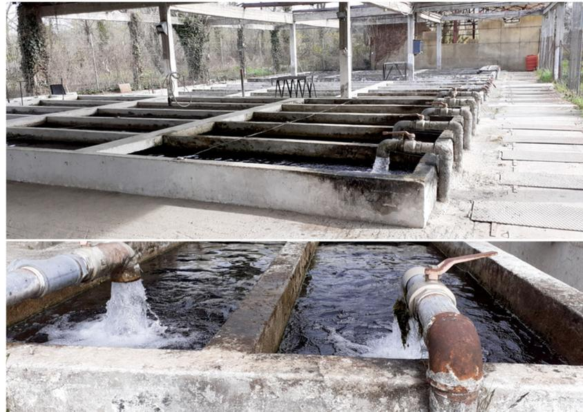
**Figure 1.** Concrete raceways built on the flow through of a small river in Pella, Greece, utilized in rainbow trout farming.
