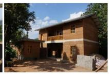
**Figure 7.** The reconstruction of Ma'anqiao Village in Sichuan Province takes advantage of the improved traditional rammed earth technique.
