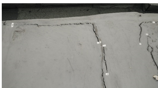
(a) Cracking
