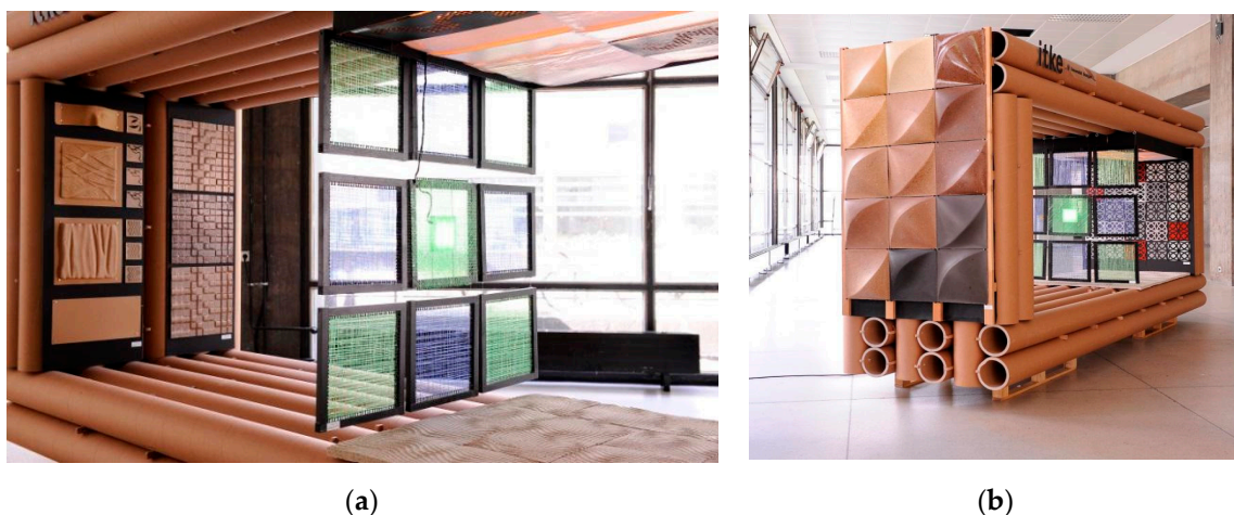
Figure 7. (a) Interior cladding applications and hanging partitions of the Eco-Pavilion (left to right): Vacuum thermoformed biocomposite prototypes, hanging partition wall from recycled plastic bottles; (b) Exterior cladding application with free-form facade panels. © BioMat/ITKE—University of Stuttgart. Photos: Miklautsch.
