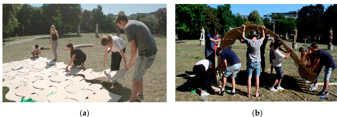
Figure 6. (a) Simple horizontal stacking by pushing modules into each other; (b) Erecting the pre-mounted pavilion by manual bending, and latter fixation with the curved foundations. © A. Coban and V. Ivanova; BioMat/ITKE—University of Stuttgart.
