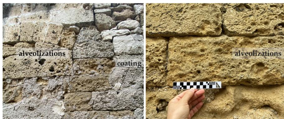
**Figure 1.** Building in Bari (Italy) realized with Gravina Calcarenite stone. It is appreciated features induced by material loss like alveolizations.
