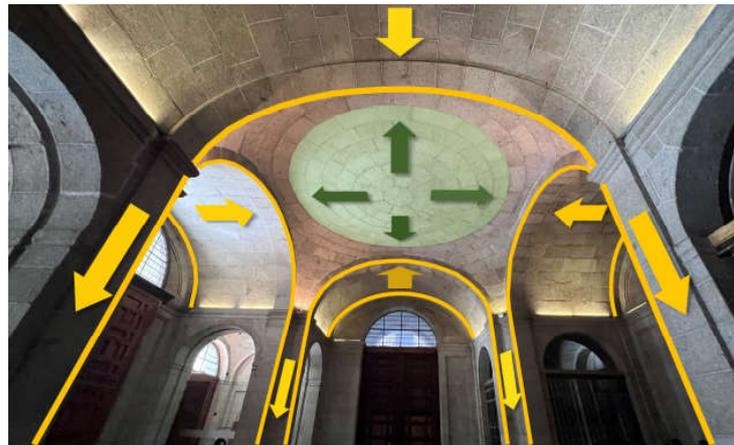
**Figure 15.** Schematic representation of the pressure transmission from the planar vault to the lateral curved vaults and the lateral walls (graph by author).
