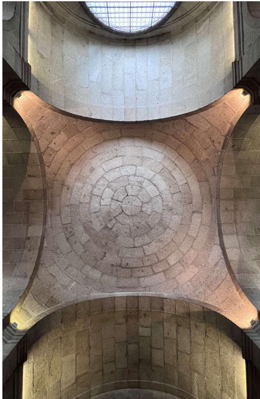
**Figure 9.** Photograph of planar vault taken from the ground (photograph by author).
