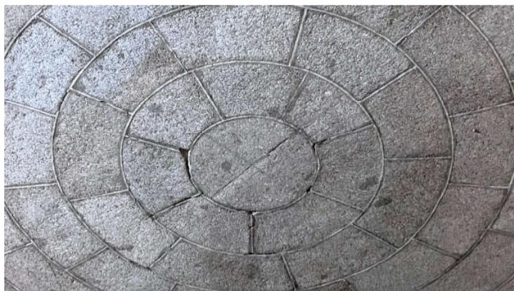
**Figure 12.** Detail of vault centre, with keystone formed by two symmetrical voussoirs (photograph by author).
