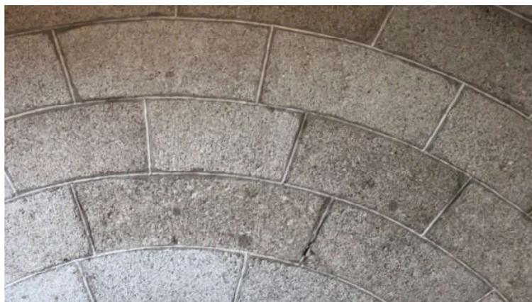
**Figure 13.** Detail of voussoirs that make up circular rings of planar vault (photograph by author).
