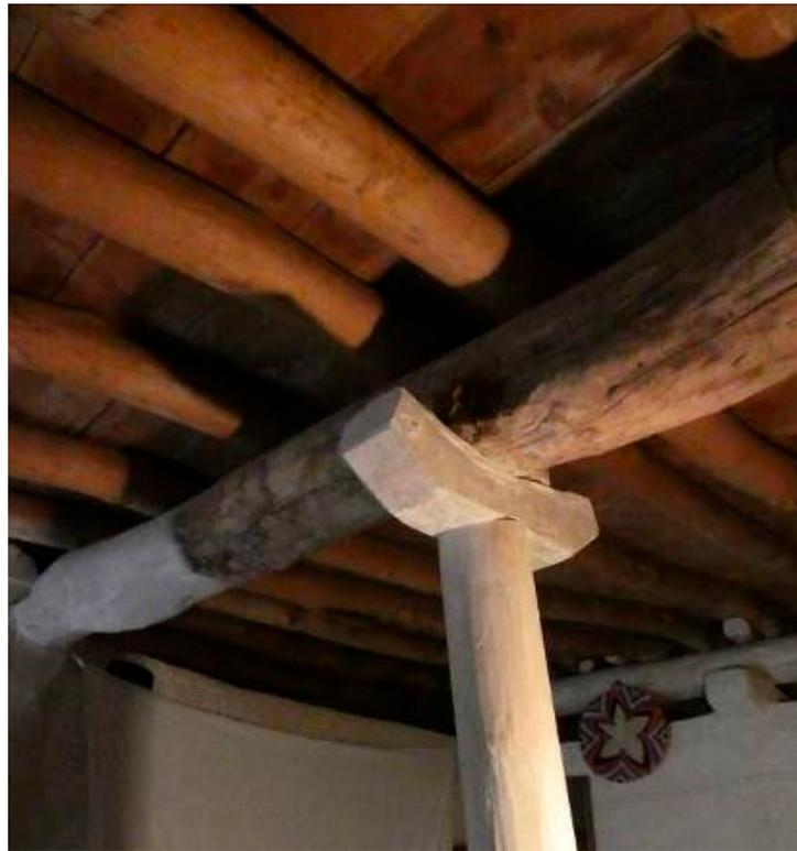
**Figure 6.** Wooden post holding primary and secondary wooden beams. Source: Author (2018).
