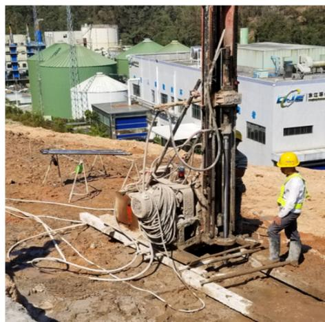
Figure 14. Lifting drill pipe during jet spraying.
