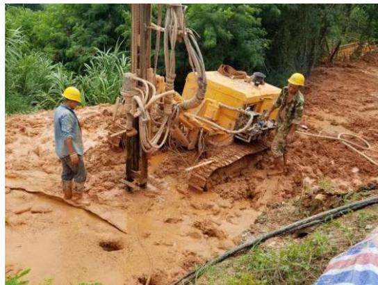
Figure 13. Pilot drill rig drilling.
