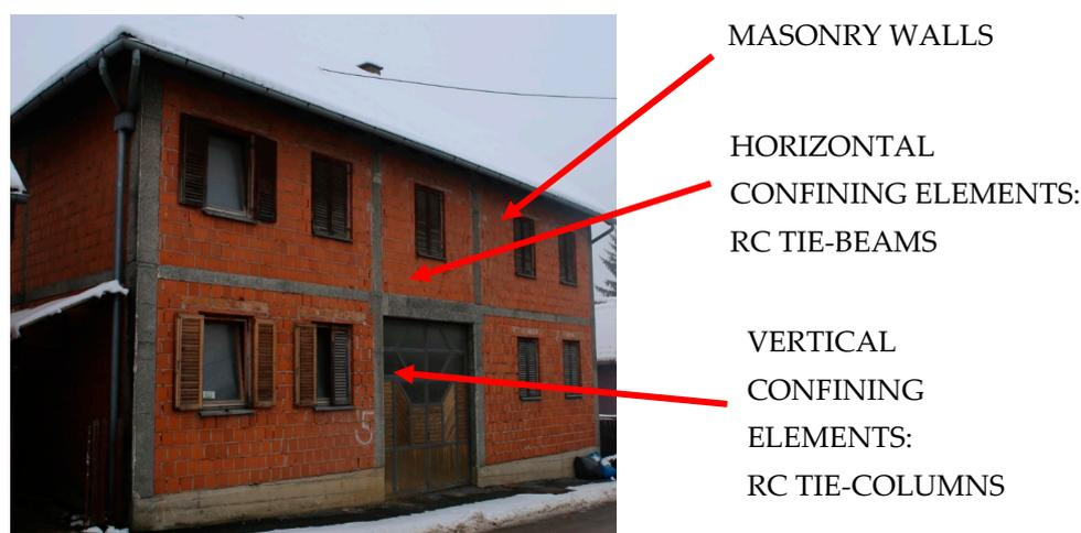
**Figure 1.** Key components of a typical CM building from the Balkan region (Petrinja, Croatia).
