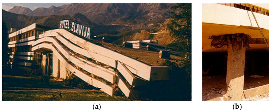
**Figure 6.** Collapse of the “Slavija” Hotel buildings in Budva due to the 1979 Montenegro earthquake: (a) a collapsed block and (b) column damage detail (credit: B. Petrović/SUZI-SAEI).
