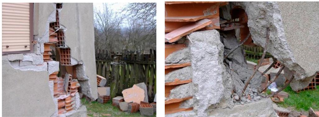
**Figure 2.** Rural single-family CM building damaged due to the 2010 Kraljevo, Serbia, earthquake, showing a failure of the RC tie column at the ground-floor level.
