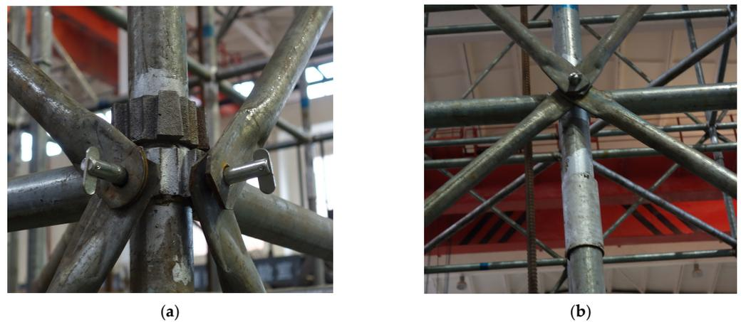
**Figure 3.** Detail of rod-end connection. (a) Connection of upright rods with horizontal rods and diagonal rods. (b) Connection of upright rods.
