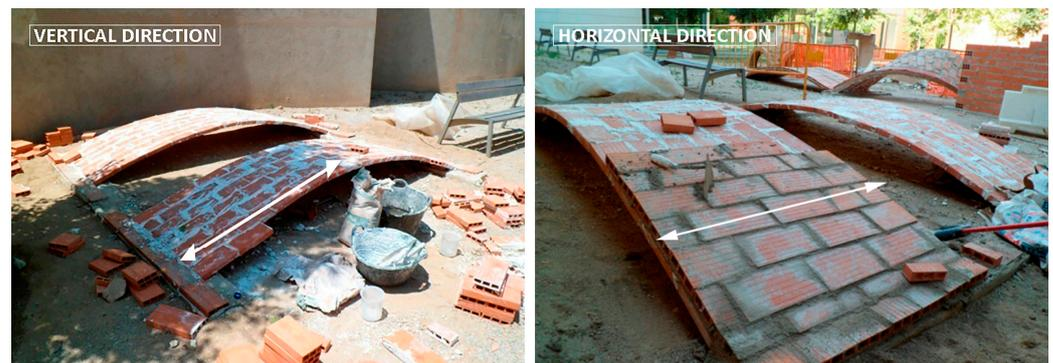
**Figure 2.** Construction of the vault: (left) first layer; and (right) second layer.
