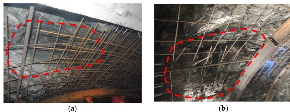
Figure 13. Image showing a failure in the surrounding rock of the Qinling tunnel: (a) left arch and (b) left side wall.
