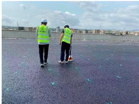
**Figure 9.** Compaction uniformity inspection.
