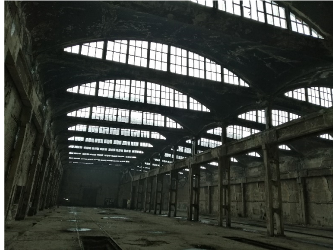
Figure 21. Ilja Doganoff. Railway Sheds of conoidal shape and semicircular clerestories in Bulgaria (1958). Source: Author.
