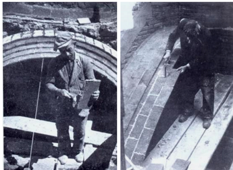
Figure 2. Illustration of Truño's book (2004). Traditional process of execution of a tile vault.
