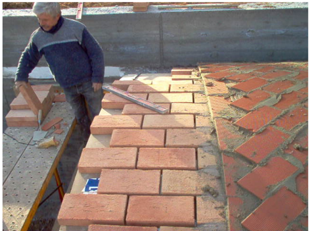
Figure 6. Contemporary process of execution of a tile vault. c. Gabriel Barbeta.
