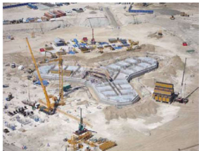
Figure 7. Tower raft foundation plan and photo of raft construction. Source: [6].
