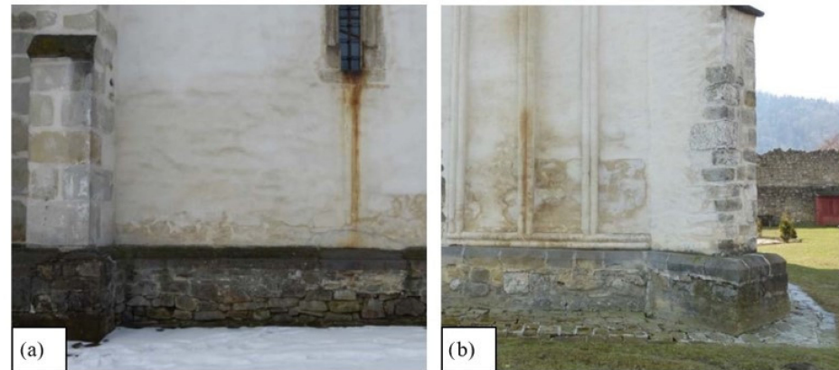
Figure 5. Examples of degradation patterns in the church of the Nativity of the Blessed Virgin Mary: (a) darkening due to rising damp in the façade, (b) salt efflorescence.
