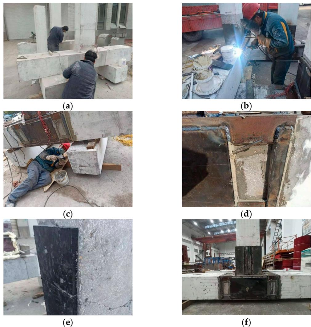
**Figure 4.** Main retrofitting processes on the pre-damage specimens: (a) grinding and cleaning; (b) positioning and welding of steel sleeves; (c) seam sealing; (d) injection of adhesive; (e) glued viscoelastic pads; (f) retrofitted specimens.
