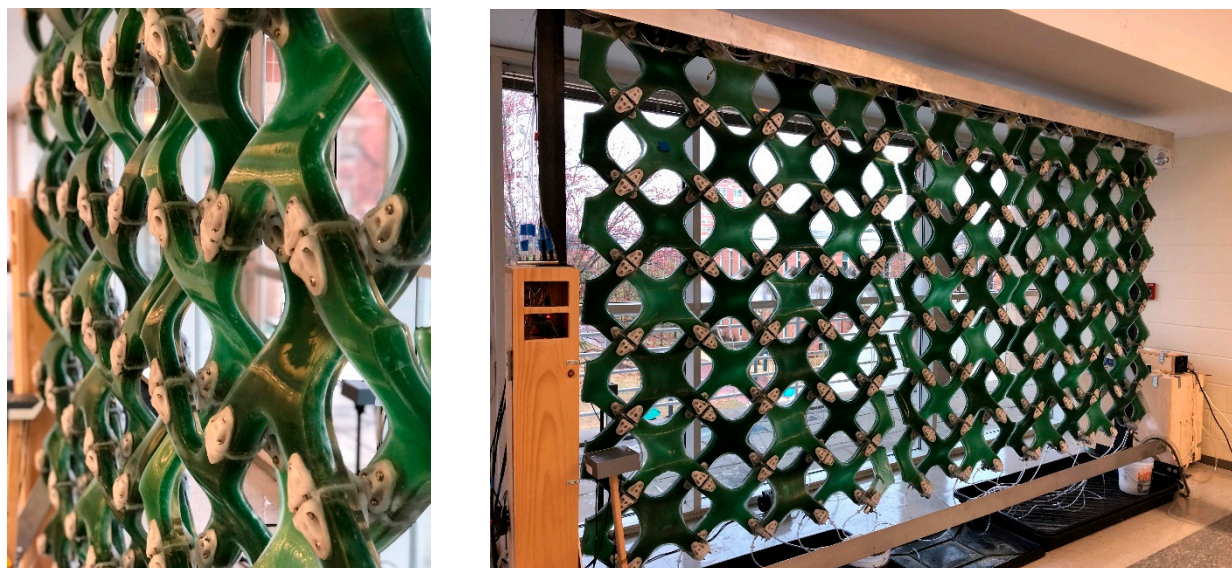
Figure 1. The microalgae façade in the creativity study is composed of a network of interlocking bioreactors filled with spirulina, blue-green microalgae.
