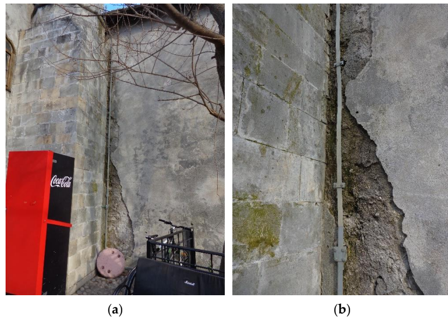
Figure 6. Plaster spalling along the vertical joint between the minaret and the mosque building (a) view (author's photo, 2023). (b) detail, (author's photo, 2023).
