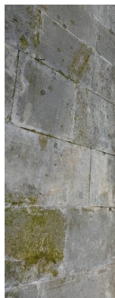
Figure 5. Biological attack at the base of the minaret (author's photo, 2023).
