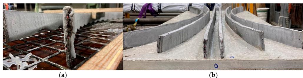
**Figure 8.** Manufacturing and assembly of the demonstrator: (a) ExCRC web assembled on grid of top slab and (b) completed ribbed slab.
