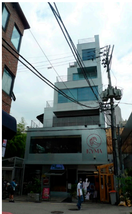
Figure 12. The form of Building 654-12, regulated by the slant line for daylight and for facing road, taken and drawn by author.
